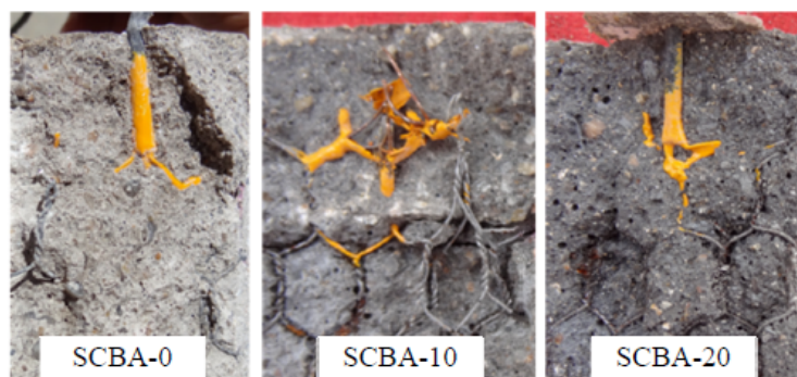
Fig. 6 Aspect of the wire-mesh connection in autopsied slabs after 2000 days of exposure in the simulated marine environment (one slab for each mortar mixture).
